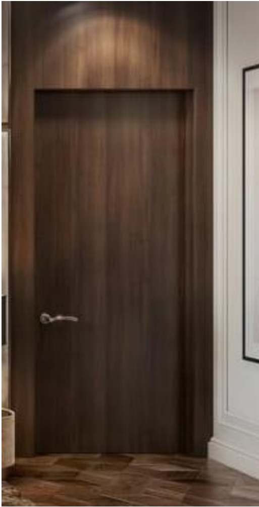
DOOR CHOWKHAT/DOOR FRAME TO BE TOPPED WITH WOODEN PANELING CONVENTIONAL DOOR FRAME NOT VISIBLE
